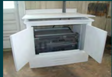
Cabinet fabricated and installed for USCG battery in kitchen
