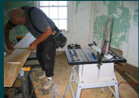
Siding replacement and USCG Bathroom dismantlement
