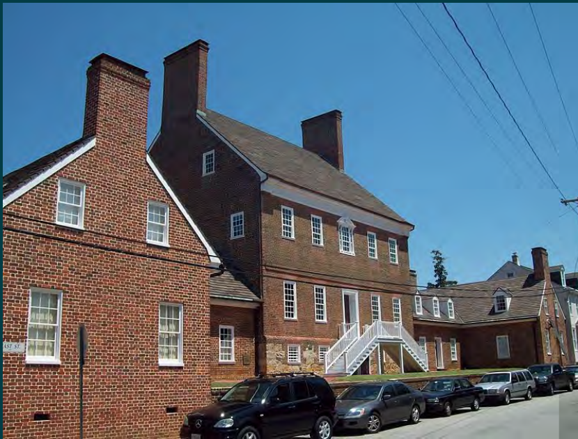
Main façade of the Brice House facing onto East Street
